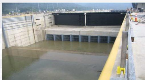
In Chamber Longitudinal Culvert System (ILCS) (Fig. 4.16)
