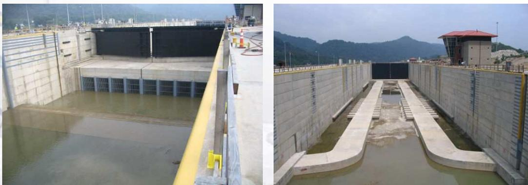
In-chamber Longitudinal Culvert System (ILCS) – Marmet Lock (Fig. 4.16)
